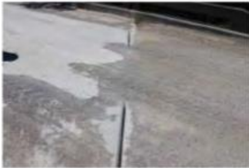
Image of structure
