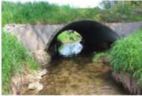
Image of structure
