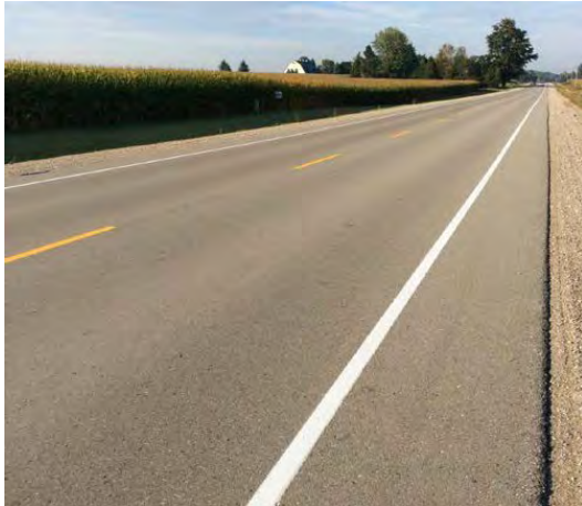
Image B.1 Rural Road with a PCI of 92.9 (Excellent)
