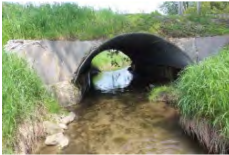
Image of structure
