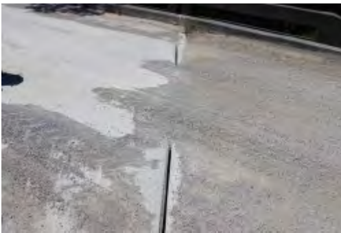
Image of structure
