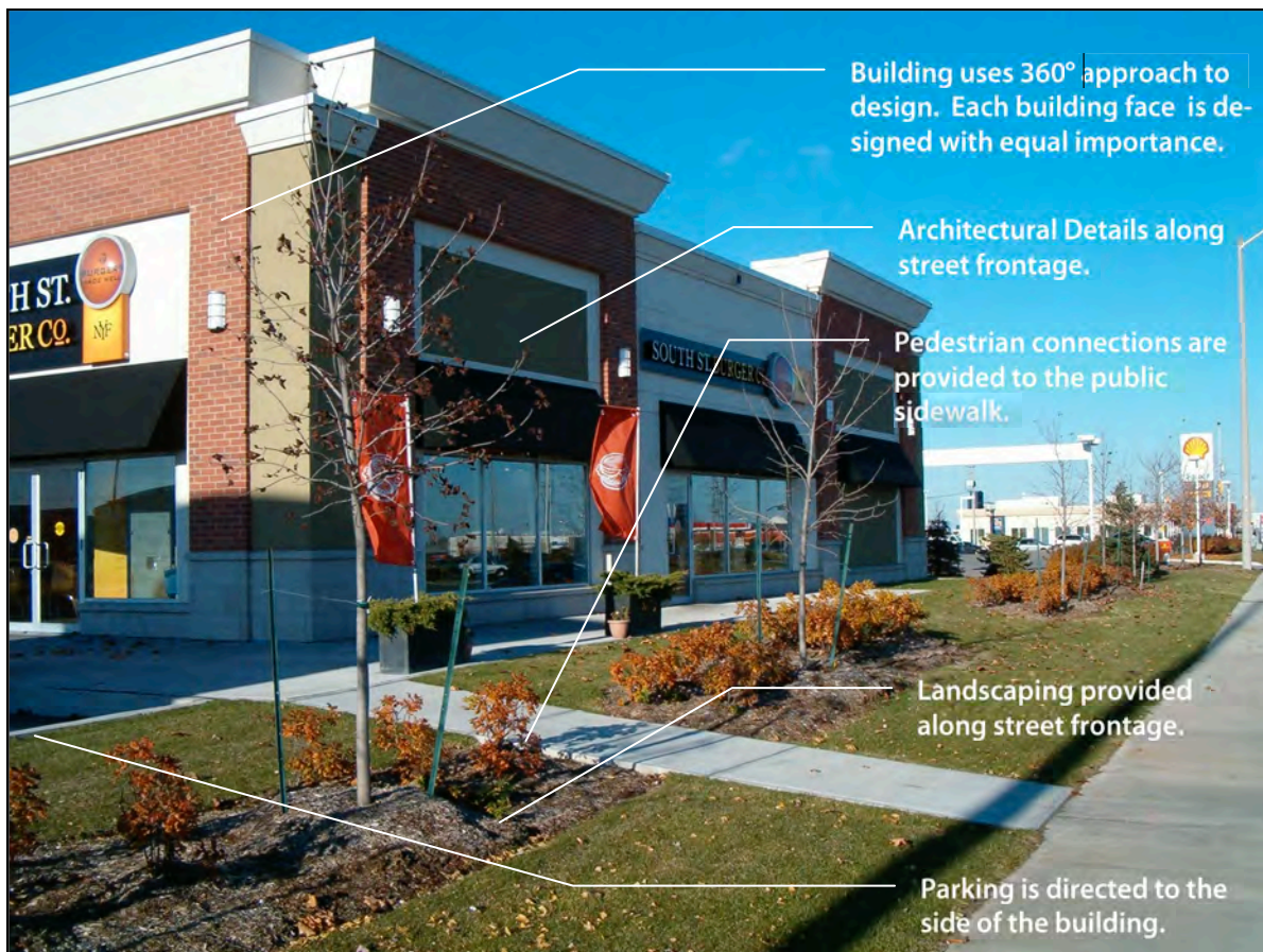
While more of an urban example, the above photo illustrates elements of good commercial design.
