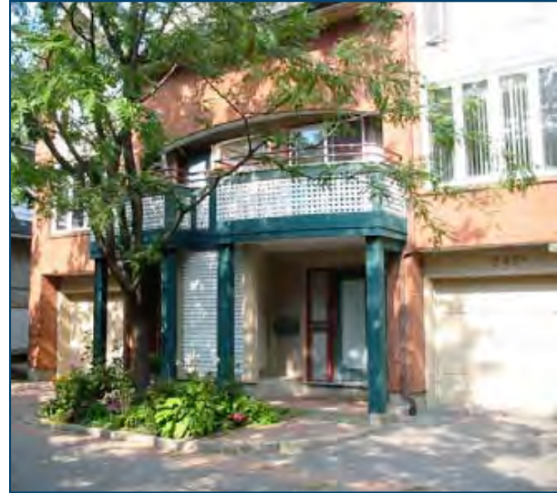
Ground floor apartment units are encouraged. Barrier free access should be provided to multi-unit developments.
