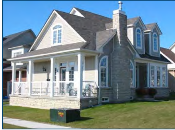
The massing of this building is broken up by windows, dormers, and the chimney projection. All of these elements add visual interest to the design of the dwelling.
