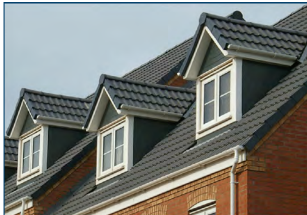
Architectural details such as dormers help to visually break up massing and rooflines.
