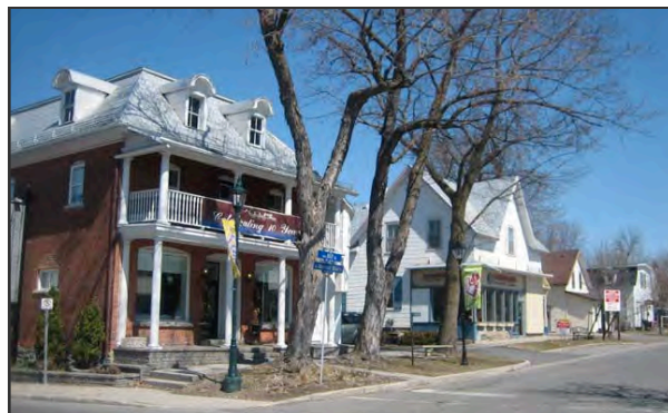
New development in the Village Cores should ensure adequate room for pedestrians, landscaping and/or street furniture.
