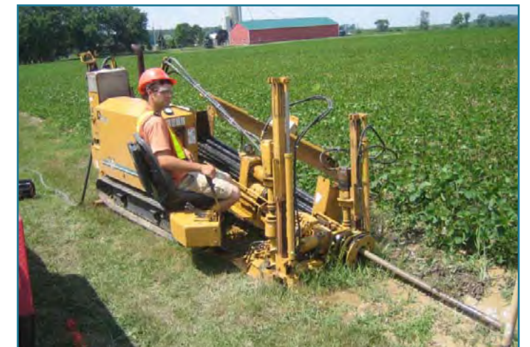
Quadro directional boring
